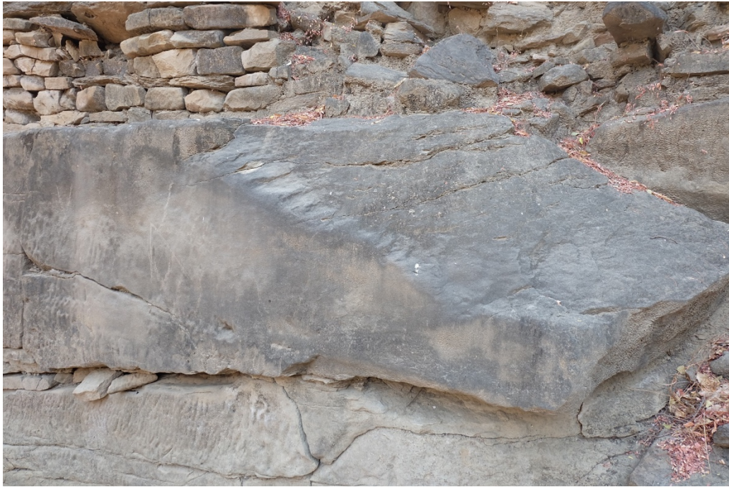
Fig 26. Symbolic (non-functional) stair carved into the sandstone bedrock of the east wall. Source: Gyles Iannone
