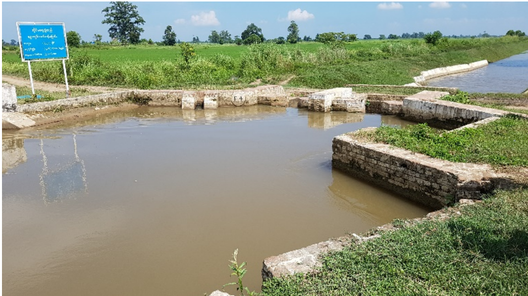
Fig 18. Contemporary choke and sluice gate along the aqueduct system at Minbu. Source: Gyles Iannone
