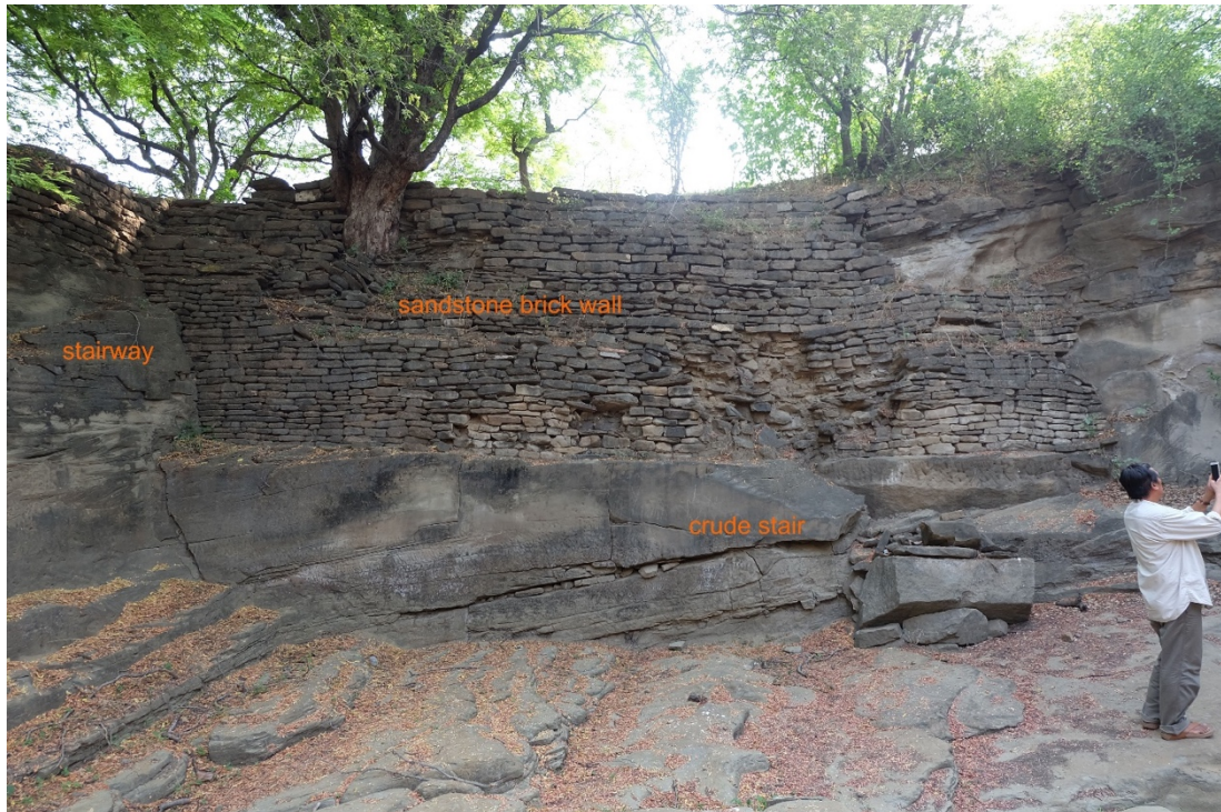
Fig 9. Northeastern stairway, symbolic stairway (crude stair), and sandstone “brick” wall enclosing the eastern side of Nat Yekan tank (note quarry scars in the lower left corner of the photo). Source: Gyles Iannone
